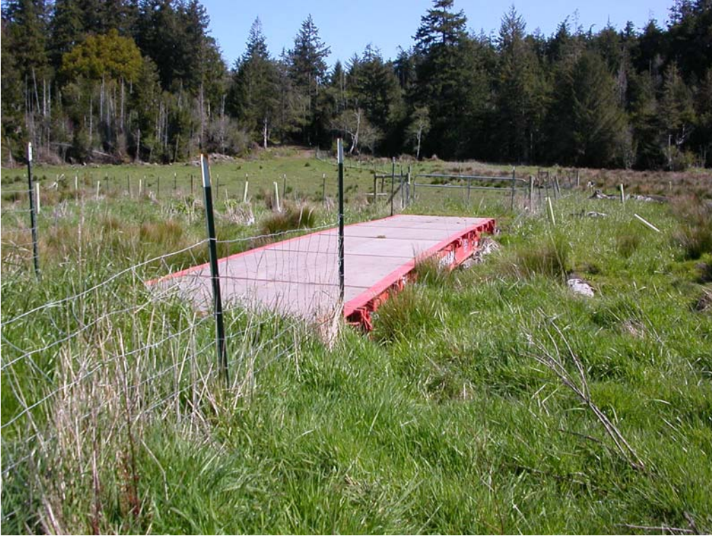
Versa-deck bridge just below pond April 2006
